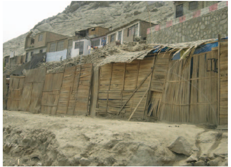
Many houses are first made with thatch; as people are able to save money over time, they rebuild with wood and eventually stone.
